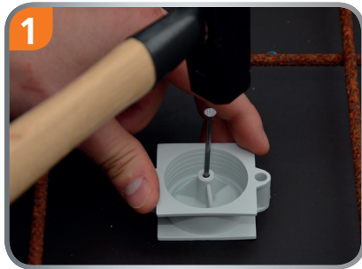
1 Nail the body of the grommet on the formwork.
